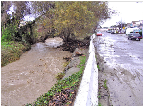
Severe rainfall has caused parts of San Pablo to experience flash floods in the past, including University Avenue next to Wildcat Creek.
