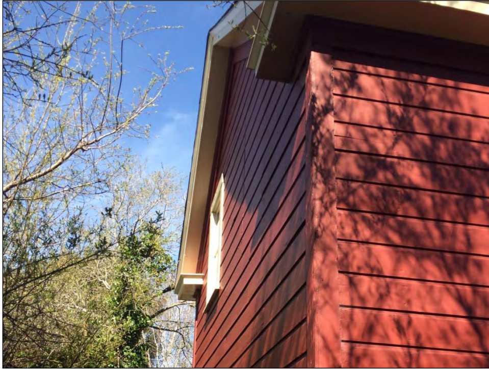
View across west-facing wall of Blume Bunk House, including patched former window location.
