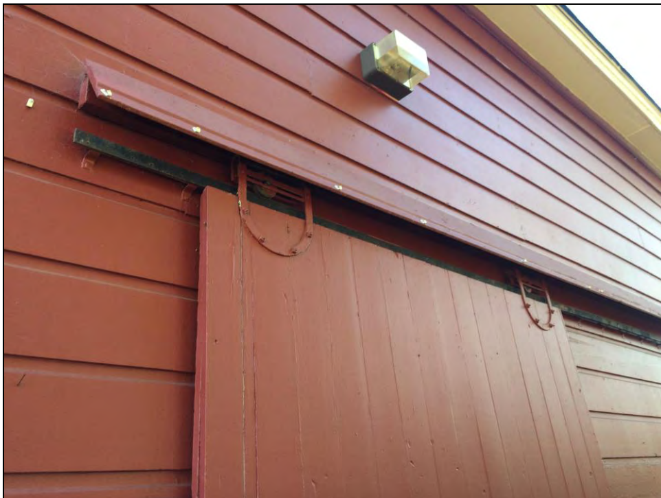
Photo 8. Detail of Blume Bunk House utility door and light fixture.
