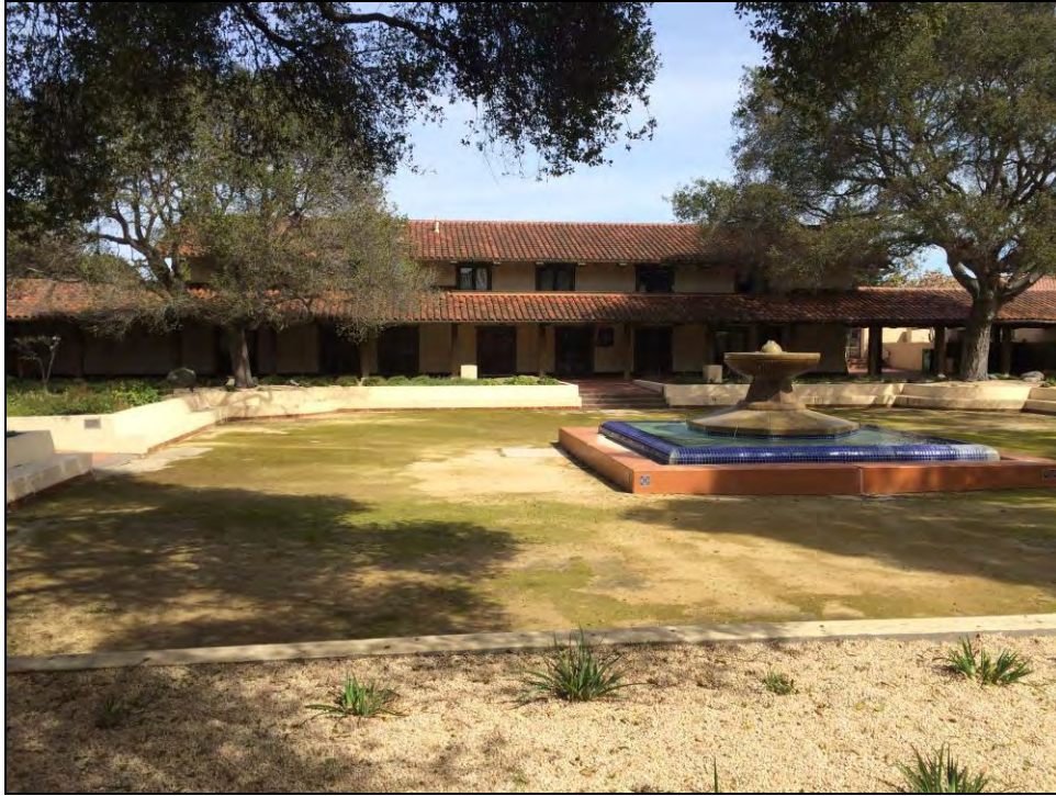
Photo 13. San Pablo City Hall Building 2, view northeast across courtyard.
