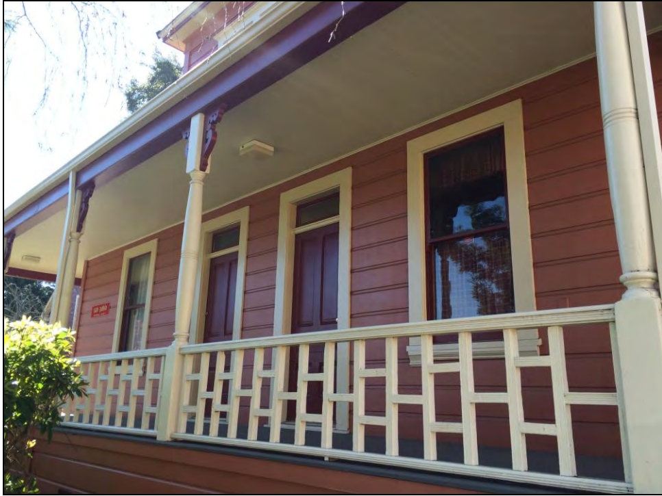
Photo 5. Blume house, view south of east-facing side.
