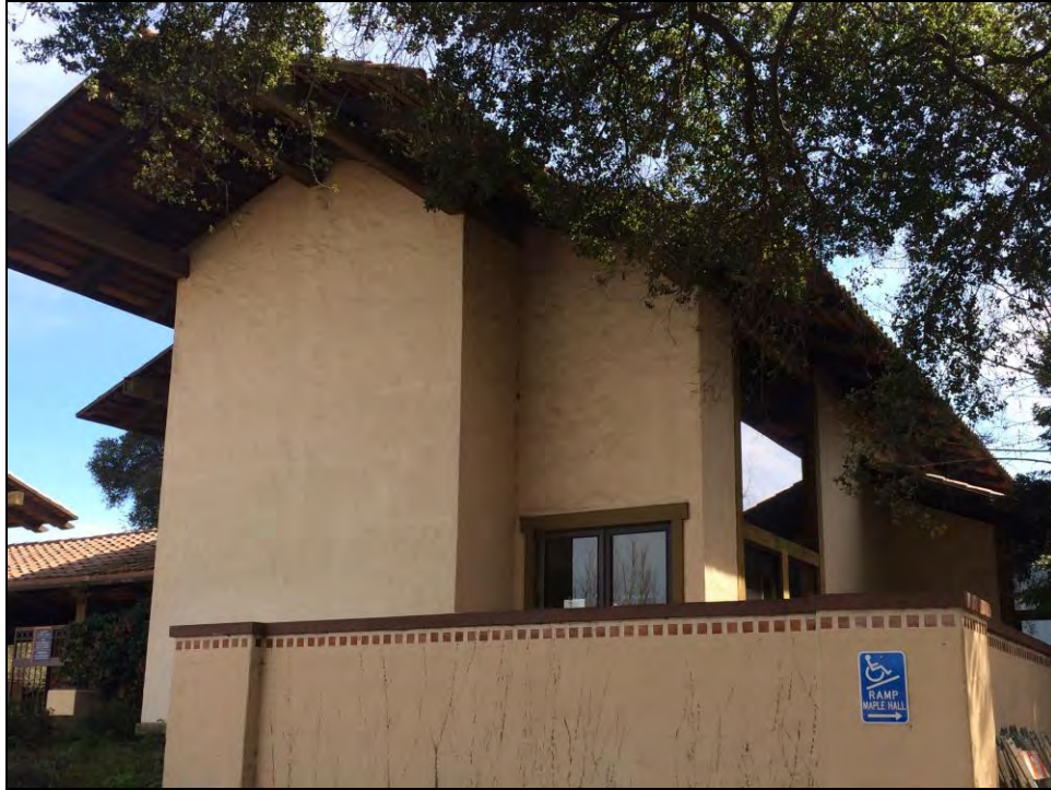
Photo 15. San Pablo City Hall Building 4, the Maple Hall Community Center, view east from outside complex.
