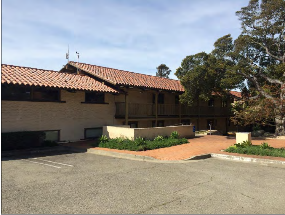
Photo 17. San Pablo City Hall Building 5, view west toward courtyard-facing side.
