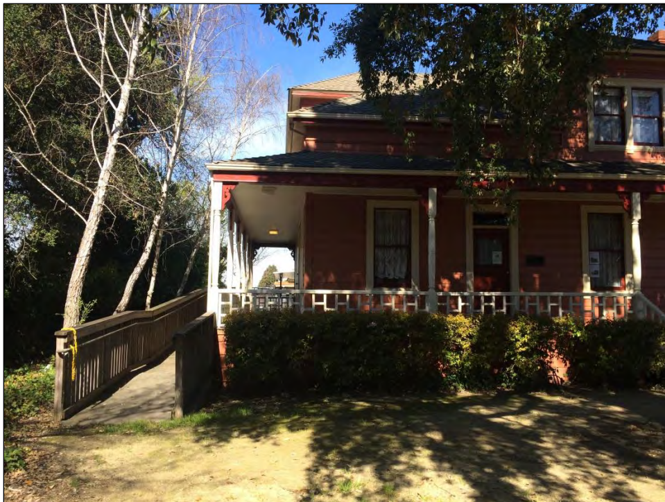
Blume house, accessibility ramp at southwest corner, view northwest.
