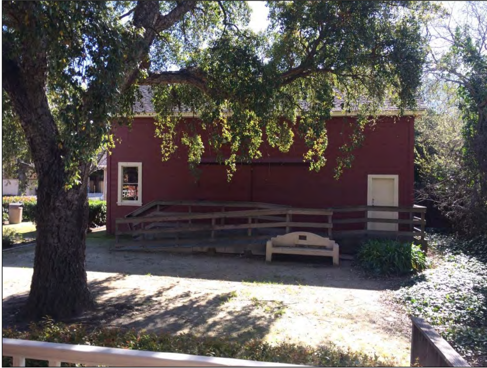
Blume Bunk House, view southeast.
