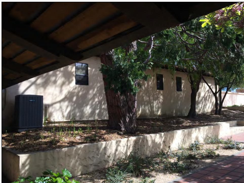
Photo 12. San Pablo City Hall Building 1, view southeast along back wall facing Building 5.
