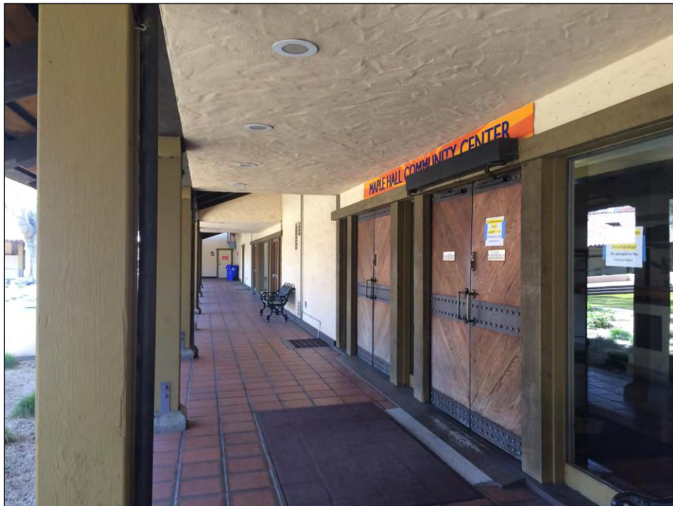
Photo 16. Main entrance of San Pablo City Hall Building 4, the Maple Hall Community Center, view southeast.
