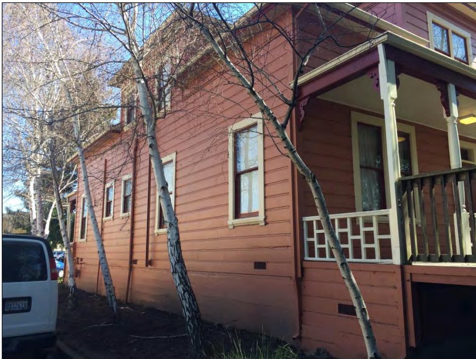
Back of Blume House, view northeast.
