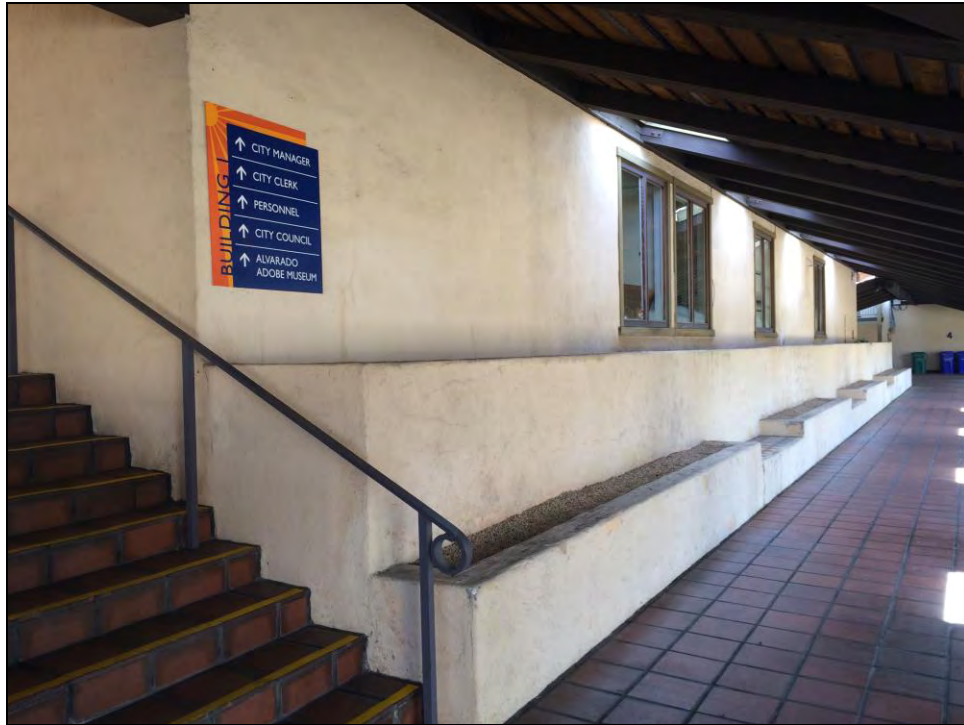
Photo 11. San Pablo City Hall Building 1, view southwest along interior courtyard-facing wall.
