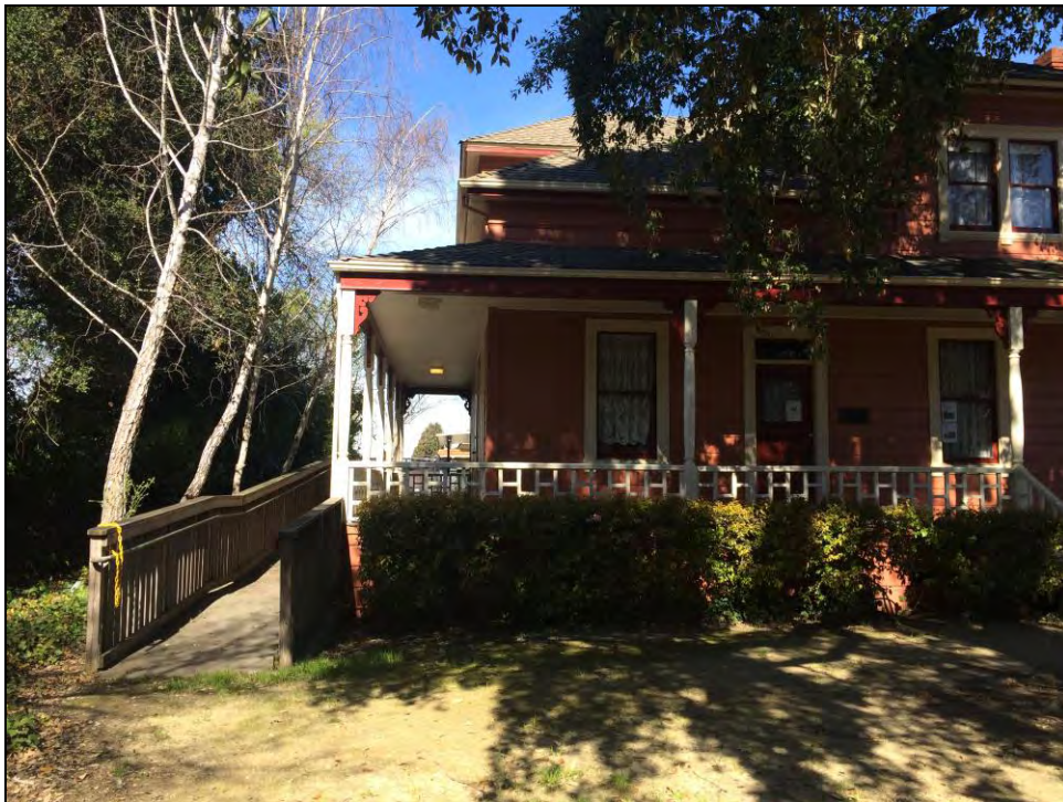
Photo 4. Blume house, accessibility ramp at southwest corner, view northwest.
