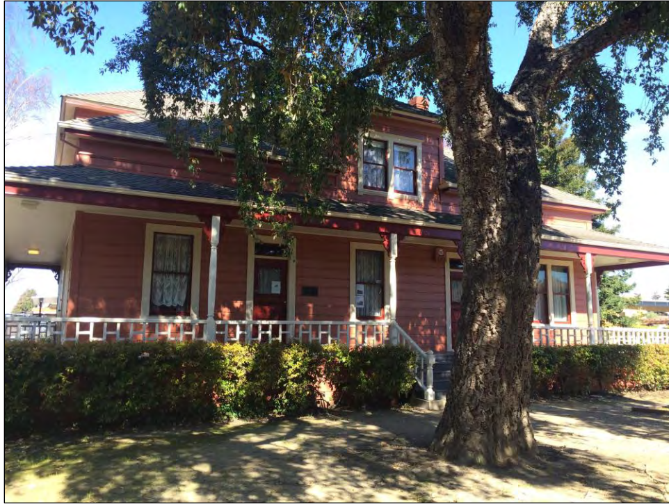
Photo 3. Blume House, view north toward main facade.
