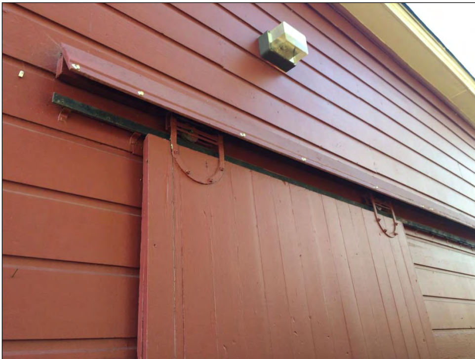
Detail of Blume Bunk House utility door and light fixture.
