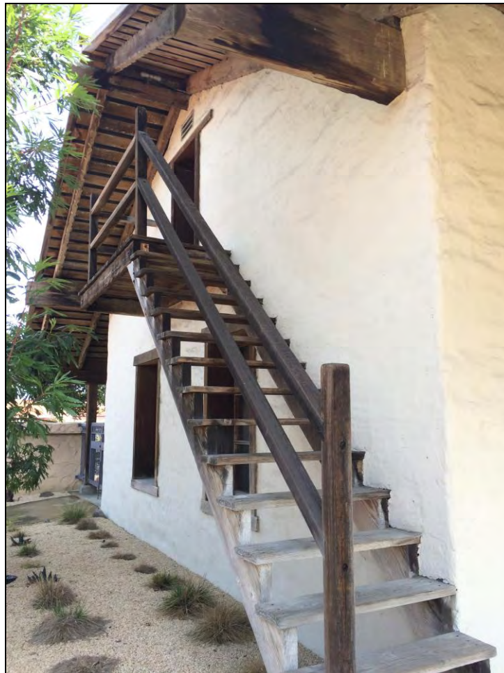
Photo 23. Exterior staircase on northern end of Alvarado Adobe Museum, San Pablo City Hall Building 7. View east.
