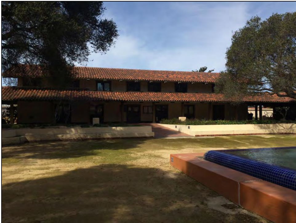
Photo 14. San Pablo City Hall Building 3, view northwest across courtyard.
